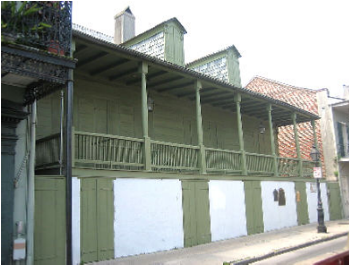
Front of 632 Dumaine Street. Taken at different times, and angles. Note all green upstairs.
